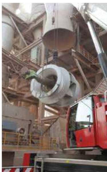
Replacement of Mill System Fan Impellar at Union Cement Factory –Ras Al Khimah
