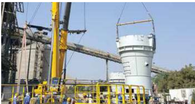
Dis - malting and Erection of Cement Mill Separator at Oman Cement - Muscat
