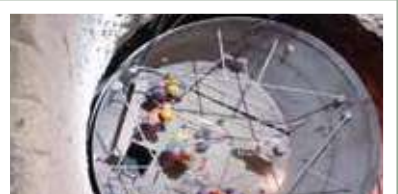
DIP TUBE REPLACEMENT AT PIONEER CEMENT INDUSTRY –AL GHAIL–RAS AL KHIMAH
