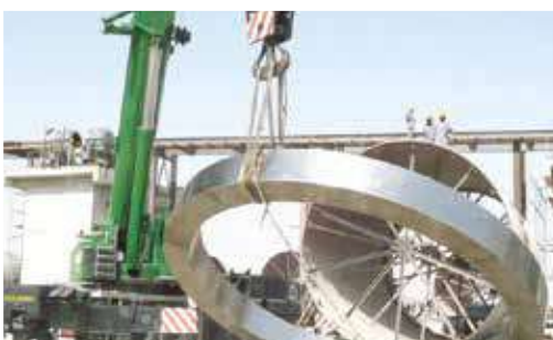
Kiln Tyre Replacement at Fujerah Cement – Dibba–Fujerah
