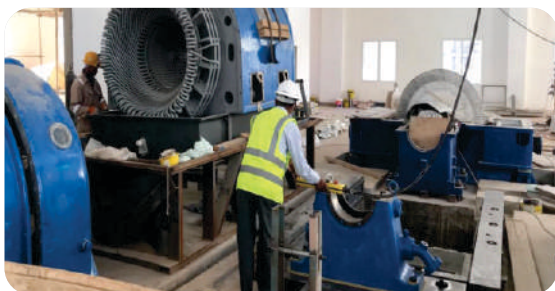
T.G Building Generator Installation
