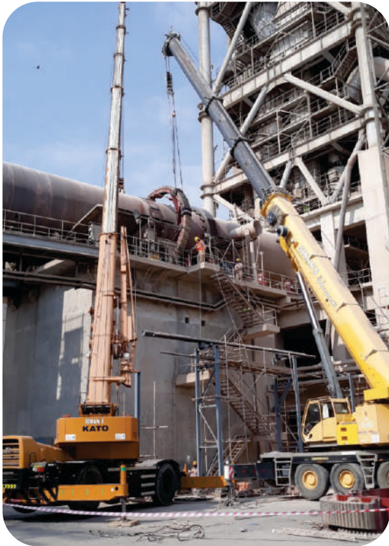
Replacement of Kiln Girth Gear Raysut Cement - Salah
