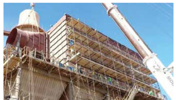
Dis - malting and Erection of Cement Mill Separator at Oman Cement - Muscat
