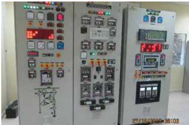
Adity Birla – WHRS –Turnine control and Automatic Synchronisation Panel
