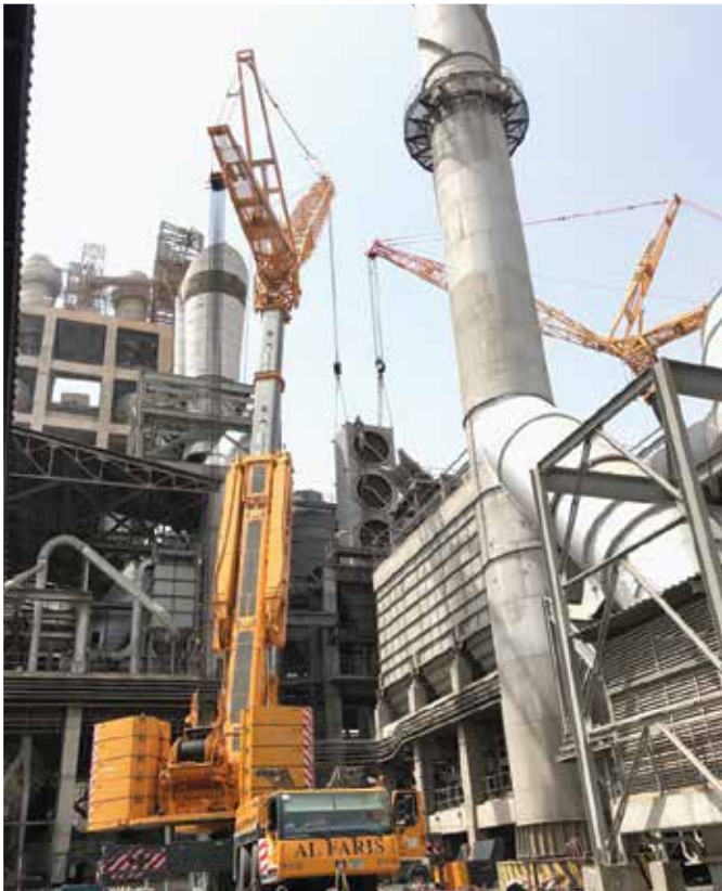
Replacement of Heat Exchanger at AGB Star Cement – RAK
