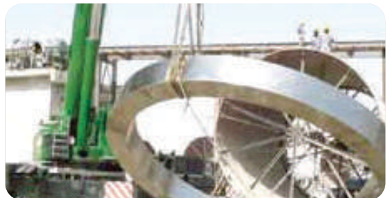
Kiln Tyre Replacement at Fujerah Cement - Dibba - Fujerah
