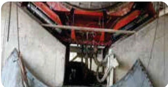
Replacement of Slide shoe Bearing at Pioneer Cement Industries LLC Al Ghail - Ras Al Khaimah
