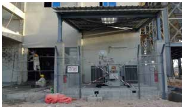
Transformers Installation
