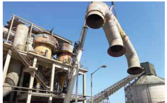
Dis - malting and Erection of Cement Mill Separator at Oman Cement - Muscat
