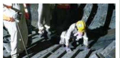
Cement Mill Liners Replacement at Gulf Cement Factory – Ras Al Khaimah
