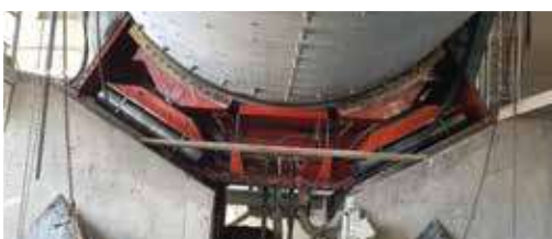
Replacement of Slide shoe Bearing at Pioneer Cement Industries LLC–Al Ghail – Ras Al Khaimah
