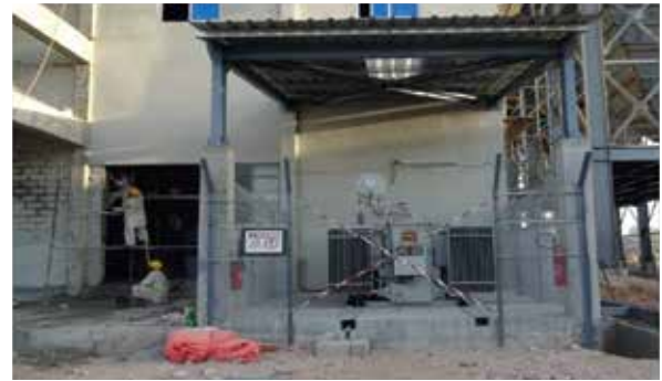
Transformers Installation
