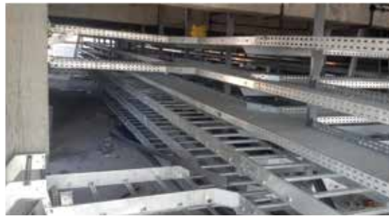
Cable Tray Installation
